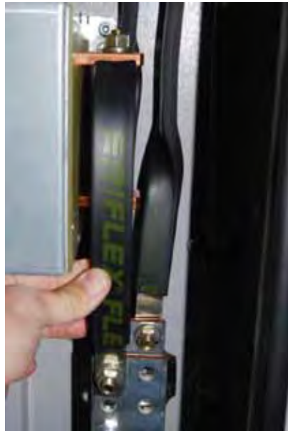
Figure 4-1 Busbars and Busbar Connection Inspection
